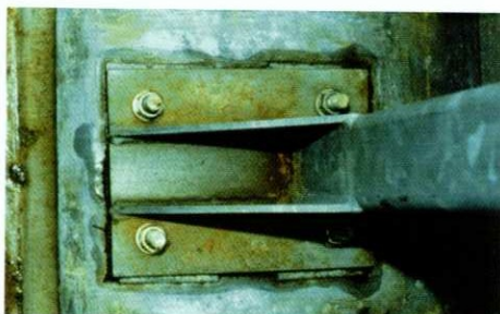
Fig 2b: This staining is superficial and can be removed to expose a sound galvanized coating beneath.
